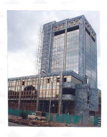
A total wall and floor area of 1,050 m<sup>2</sup> was treated using 1811 kg of *Xypex Concentrate*, 1175 kg of *Xypex Modified*, and 800 kg of *Xypex Patch and Plug*.
