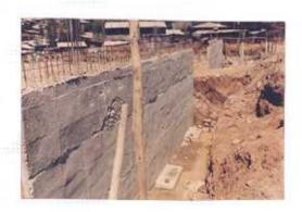
The Xypex waterproofing system was specified on this shopping centre project in order to prevent moisture in the backfill from damaging rebar and also to prevent moisture appearing on the inside faces of the walls.
